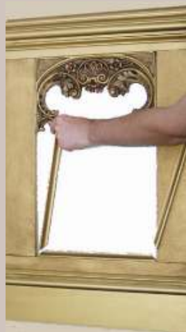
Then miter and attach the 3 pieces of inner cove molding with adhesive caulk. Top of two side moldings should be cut to 90 degrees, bottoms of cove molding cut to 45 degrees.
